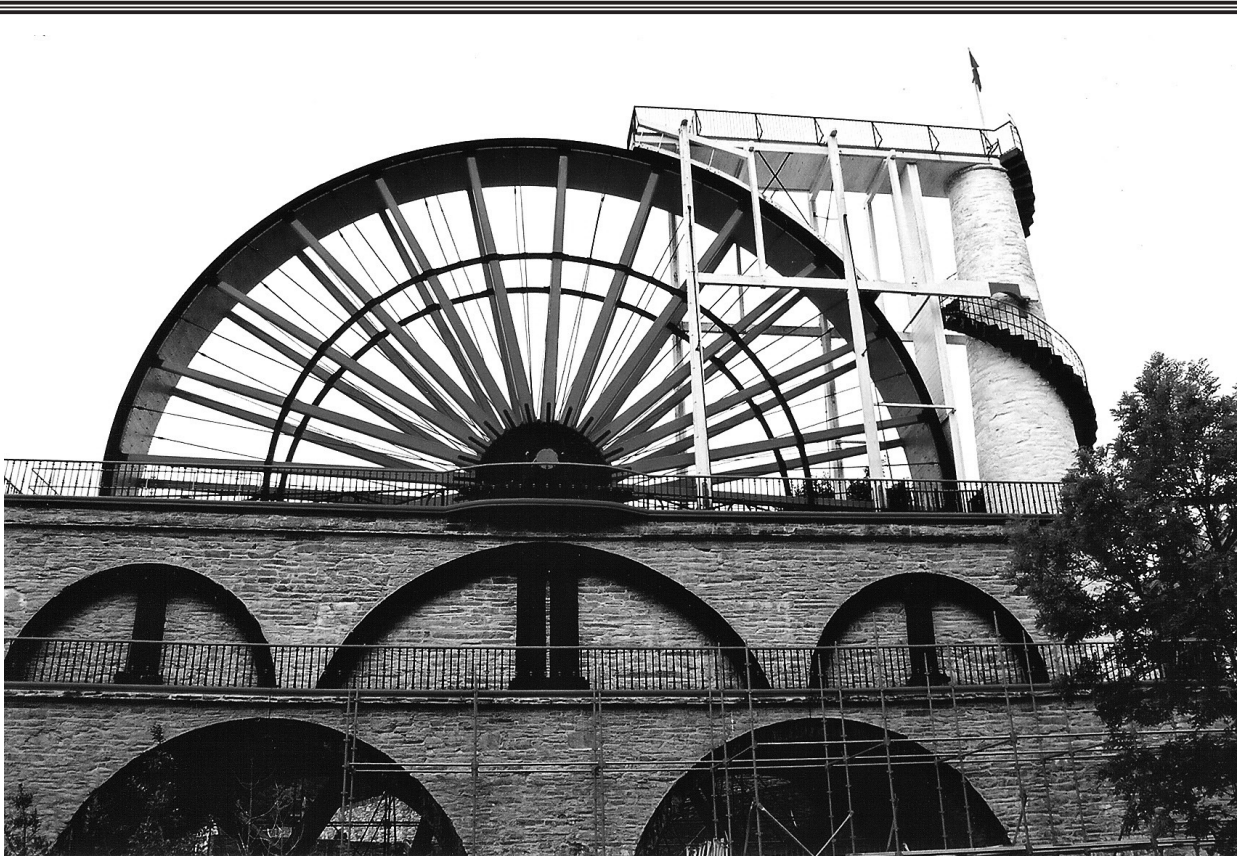
The Great Laxey Wheel is undergoing repairs
